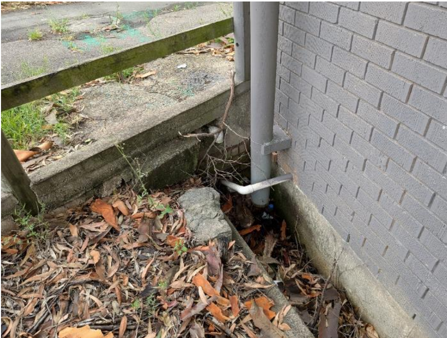
Image 6.6.1 Drainage pipes observed in north-eastern corner of the site potentially comprising asbestos containing materials.
